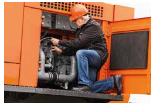
Easy access for maintenance.
