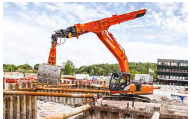
Special application excavators
